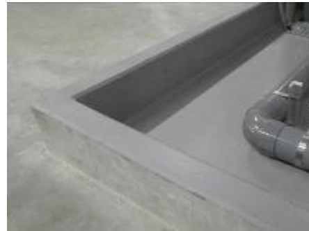
Dike (Waste Water Relay Tank)
