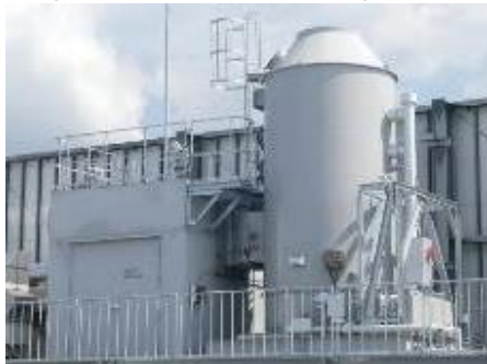
System for Cleaning Exhaust Gas
