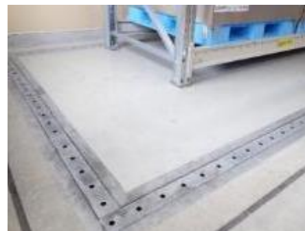
Pit to Prevent Leakage
